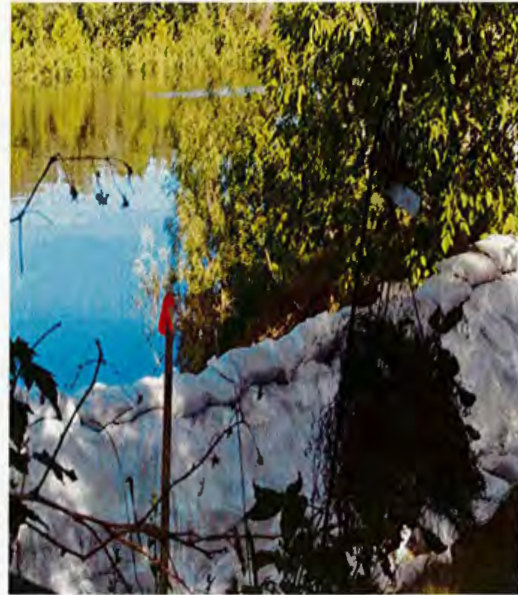
Bracken Dam, OCN 211 - Sandbagging
