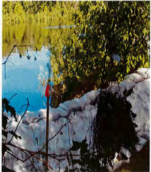
Bracken Dam, OCN 211 - Sandbagging
