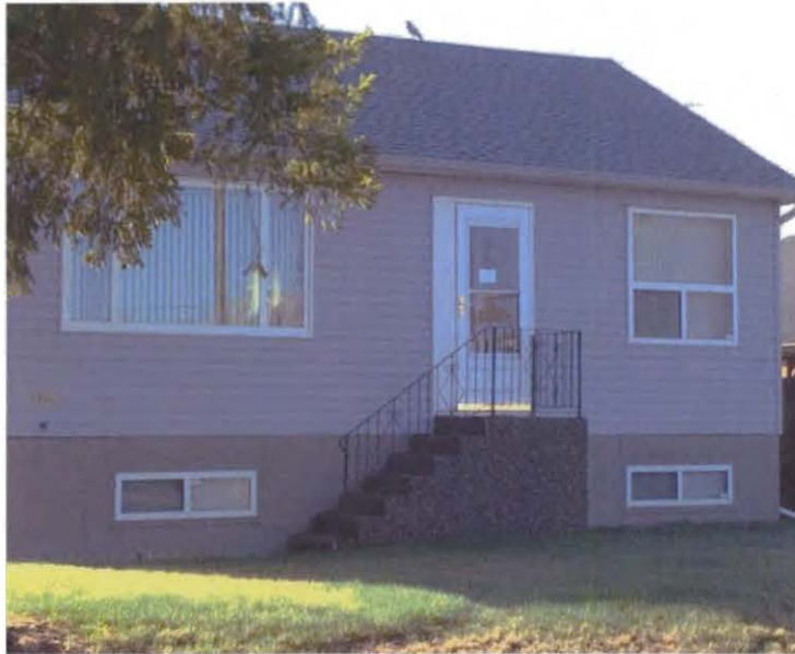
For this house, the setback from the property line is measured from the house, while the steps leading to the front door project or intrude into the setback area
